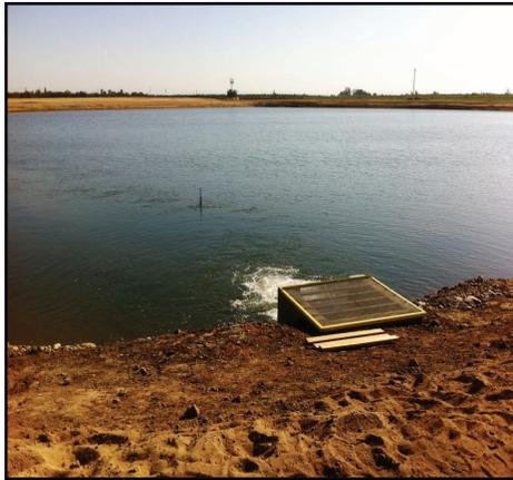
*MID began delivering water to the Cressey-Winton recharge basin in 2011. Within less than three months, MID has delivered at least 1,300 acre feet of water to the aquifer used by agriculture and the cities of Merced, Atwater and Livingston. The basin is used to assist in recharge of groundwater during years when water is available from Lake McClure.*
